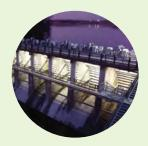
Vermilion Dam In 2020, Aqua Illinois completed \$20 million in capital improvements to the Lake Vermilion dam. Originally built in 1925 to create a reservoir and recreational lake, Aqua Illinois replaced 11 floodgates and made structural dam modifications to protect this vital water source. The project preserved the lake for the public to enjoy for future generations.
