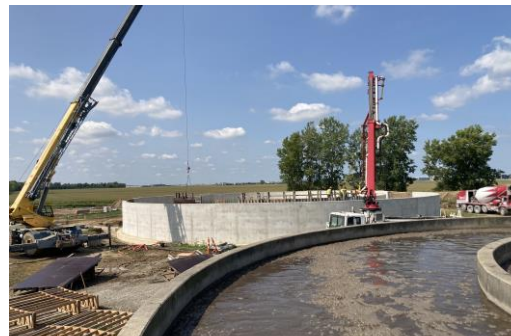
Hancock Wastewater Treatment Plant Expansion
